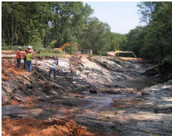
Photo 1 – Prior Excavation of Creek Bed
