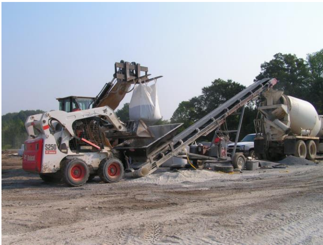
Photo 3 – Preparation of AquaBlok Blended Barrier
