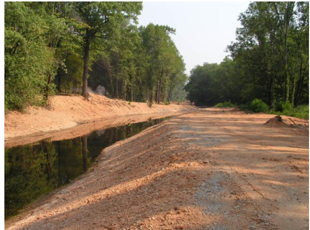
Photo 6 – Finished Creek Section After Flood Event
