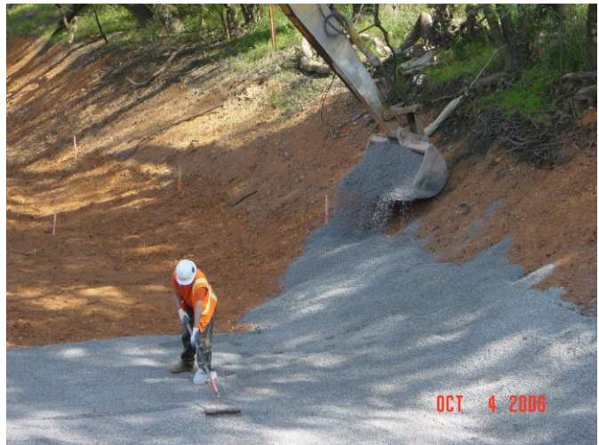
Photo 4 – Application of AquaBlok to Creek Bed
