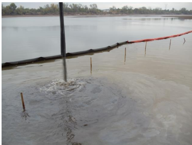
Above – Close-up of Telebelt Material Placement
