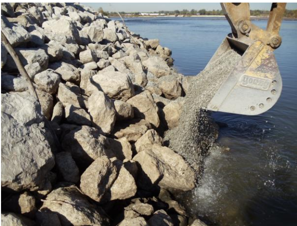
Left – Placement of AquaBlok Over Rip Rap Below – Using Blower to Distribute AquaBlok
