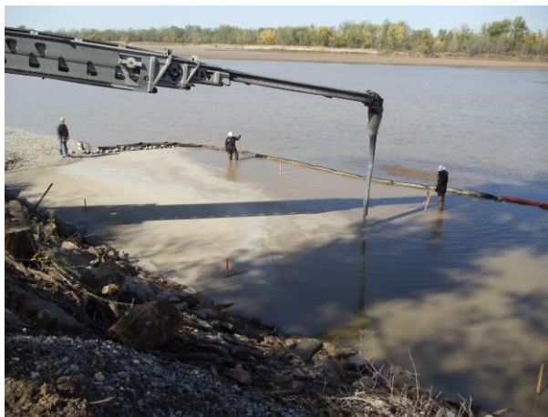
Above – Placement of AquaGate+Organoclay
