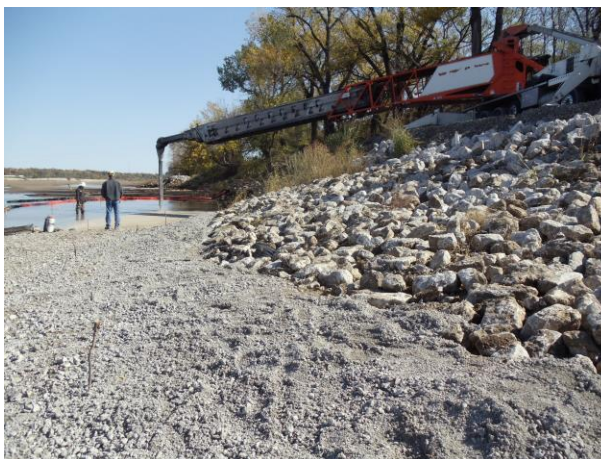
Above – View of Telebelt During Armor Stone Placement
