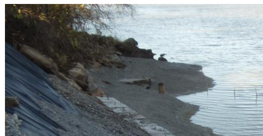
Above – Demo Debris Area - After
