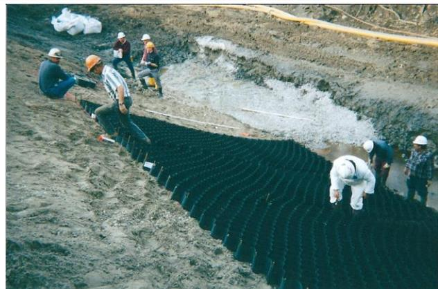
**Method of AquaBlok Placement:** Material placed directly from Supersacks suspended from a shore-based excavator (shown on previous page).
