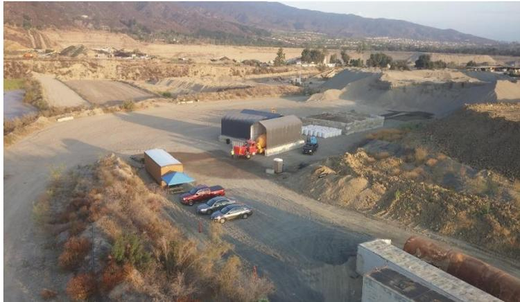
To the **right** is a photo of the AquaBlok stockpiled at the project site. After off-loading from the trucks, stacking conveyors were used to create large piles that could be covered with a high density plastic cover to protect the material from rain. It was estimated that from 1%-3% handling losses would take place due to material handling and storage losses.
