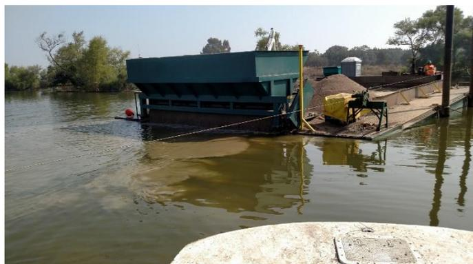
The photo on the **right** shows the material stockpile on the placement barge and the mini-excavator that was used to load the hopper.
