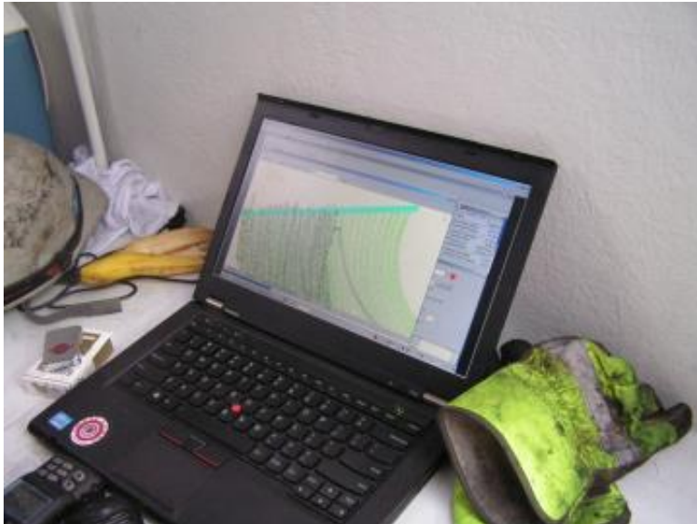
GPS quality control and documentation of placement
