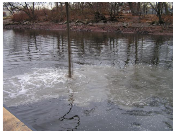
View of sand turbidity in water during placement
