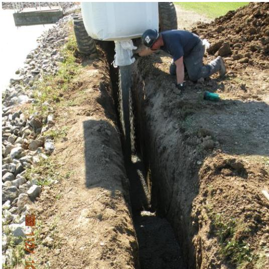
**Photo 3:** Final trench section excavated and now being backfilled with AquaBlok 3070FW(#8).
