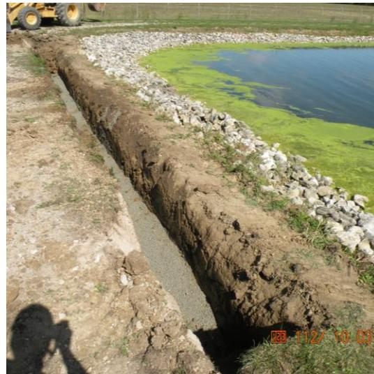
**Photo 4:** Final 48' long (approx.) x 18" wide trench cut-off wall backfilled with AquaBlok 3070FW(#8).
