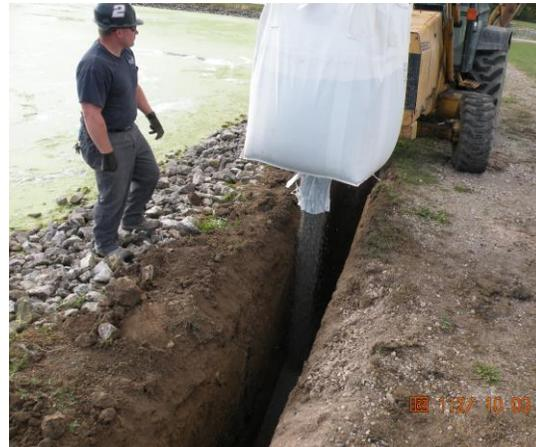
**Photo 2:** Material installed directly from bulkbags
