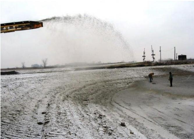
Photo 4. AquaBlok placement from a shore-based stone slinger truck. Note dusting of snow on sides of slope and top of bank, as well as the remote-controlled operator standing in basin
