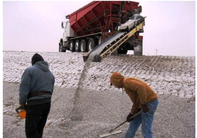
Photo 5. Shore-based stone slinger truck being controlled by operator (left). As product is placed, fine adjustments in material thickness can be easily achieved using a concrete float or rake
