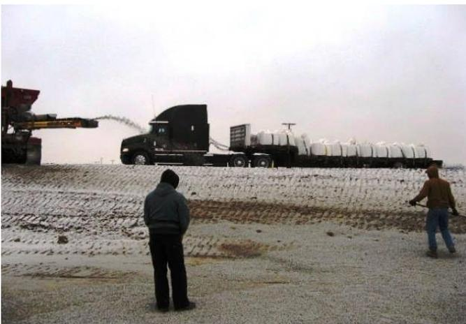
Photo 6. Delivery of a flatbed carrying ~22 tons of AquaBlok packaged in bulk bags. Note tarp has been removed to facilitate transloading into the slinger truck
