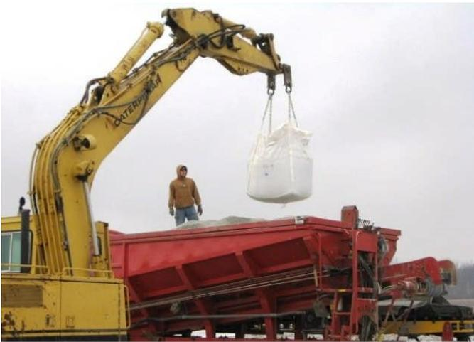
Photo 2. Transloading of AquaBlok from a bulk bag (standard shipping unit) to the bed/hopper of the application equipment - a stone slinger
