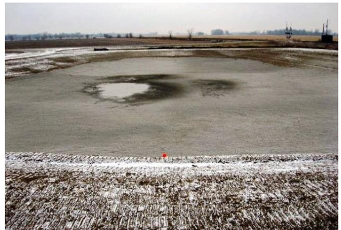
Photo 7. 35,000 square feet (0.8 acre) of basin floor newly lined with AquaBlok at 7lbs/SF (nominal 1" dry thickness). Note pooling water caused by hydration of bentonite (darkened product at center)
