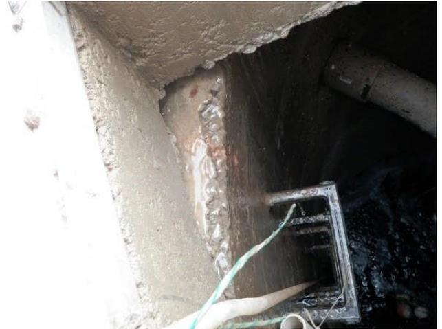
Photo 3. Leachate collection basin beneath poured concrete pad (See Photos 2-6) showing surface water flow between top of precast concrete structure and bottom of pad (compare to Photo 7).
