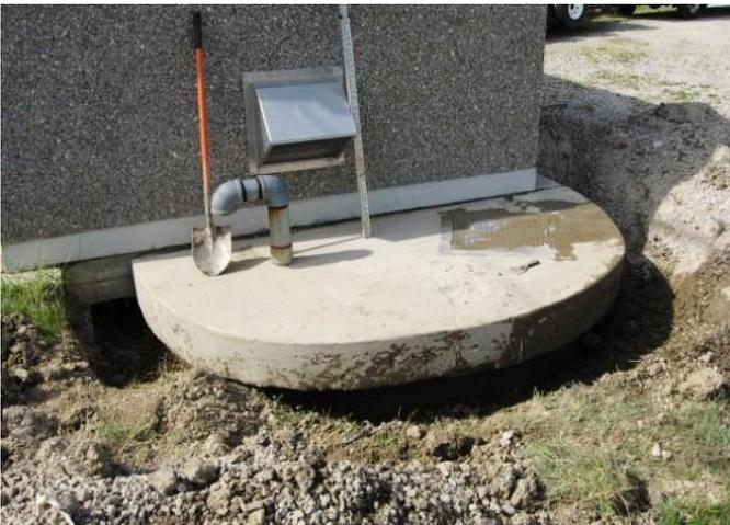
Photo 4. Excavation around concrete pad exposing seam between precast structure and pad.
