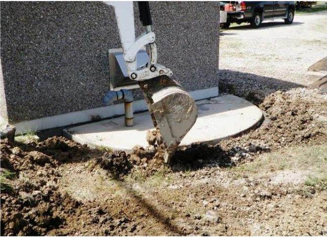
Photo 6. Placement of topsoil atop AquaBlok prior to finish grading and seeding.
