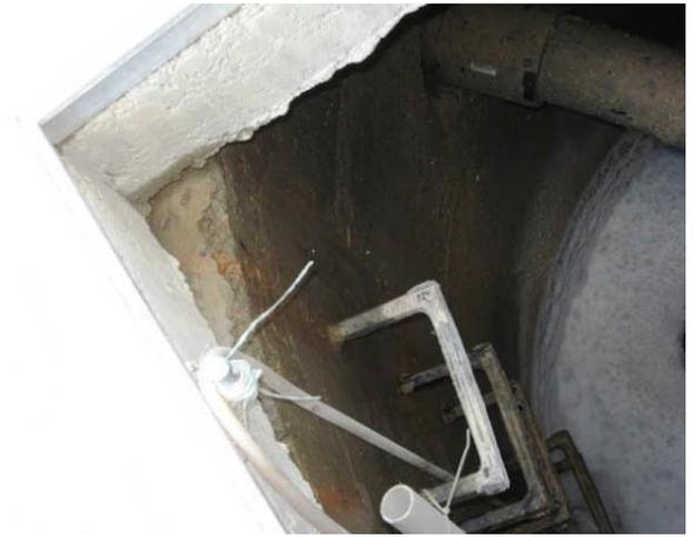
Photo 7. Leachate collection basin beneath poured concrete pad showing lack of surface water flow between top of precast concrete structure and bottom of pad (compare to Photo 3).
