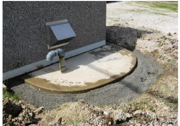
Photo 5. Apron of AquaBlok approximately 1'W x 1'D surrounding both the structure and the pad (See Photo 1 for application from bulk bag). Note product has been hydrated.
