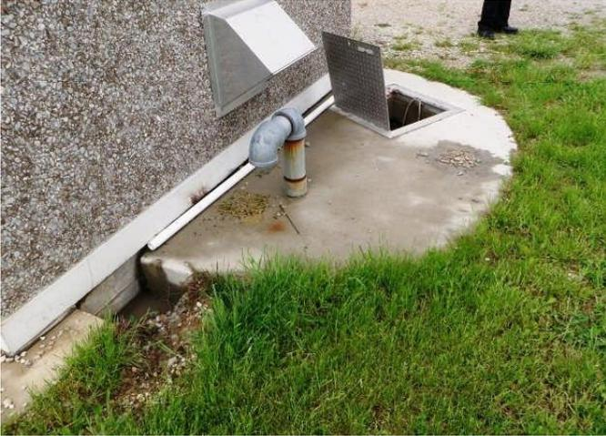
Photo 2. Poured concrete pad adjacent to leachate collection pump station. Collection basin (See Photos 3 and 7) lies beneath pad at base of disposed cell.
