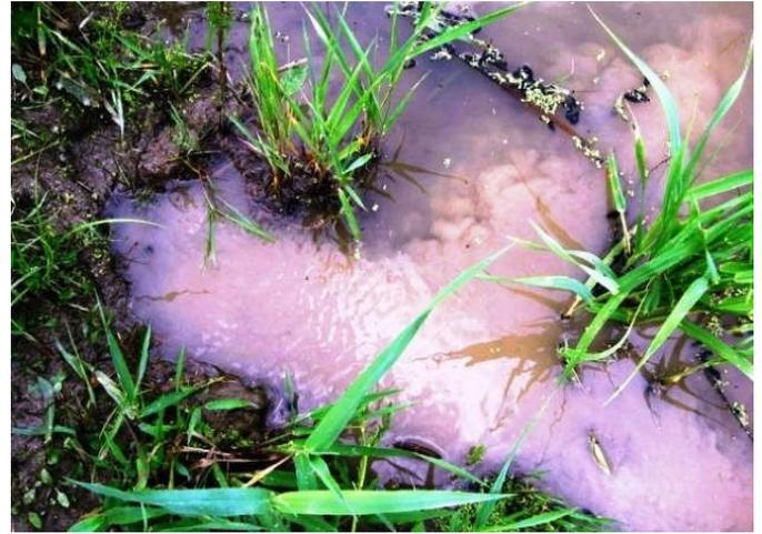
Photo 3. A top-down perspective of the water upwelling on the “back side” of the earthen berm – in the environment which was intended to be moist (not inundated).
