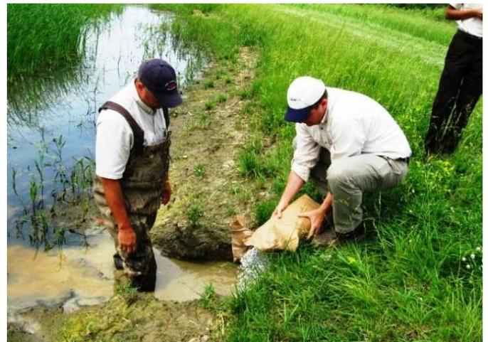
Photo 5. Manual addition of AquaBlok from a 50lb bag.
