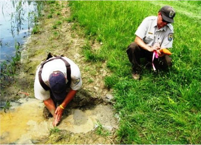
Photo 6. Active hydration of AquaBlok (five bags of 250lbs total) following product placement. Note technician marking location with GPS to track performance through time.
