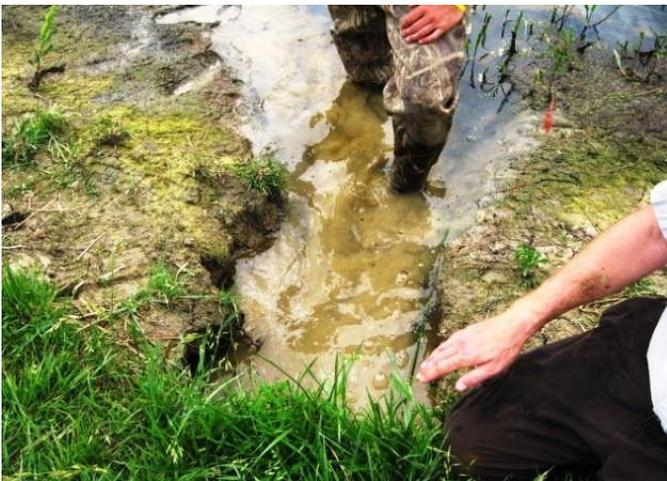
Photo 4. After closer inspection, the pathway (which measured exactly 24” wide) was determined to be the result of an improperly re-compacted trench dug to remove a remnant field tile.
