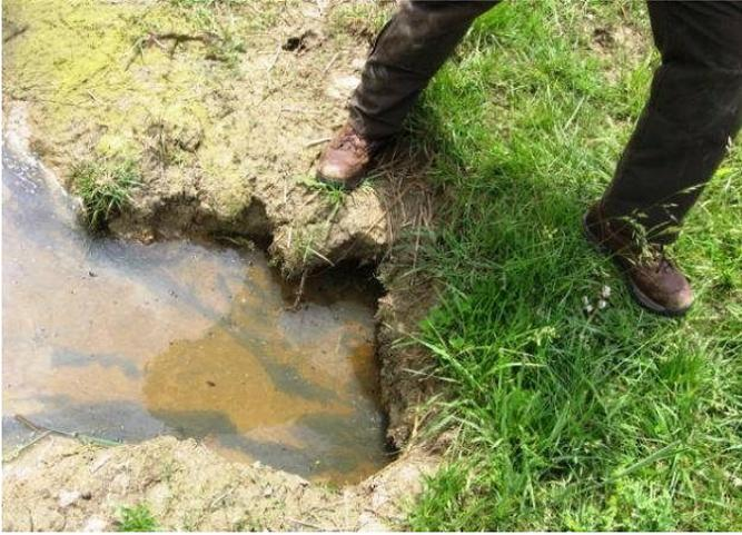
Photo 2. A top-down perspective of the breach in the earthen berm separating an inundated wetland (left) from an adjacent non-inundated wet prairie environment at drawdown (right).
