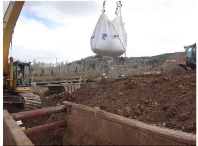
Photo 4. The excavator bringing over a bulk bag (standard shipping unit for bulk material) to the trench to be placed into the trench dam form.
