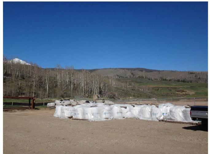
Photo 2. Storage of the AquaBlok material on site. Tarped and protected from the elements.
