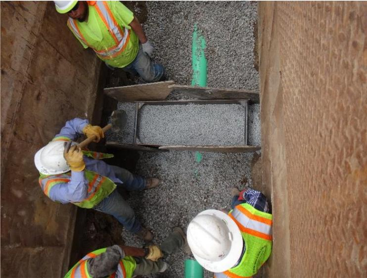
Photo 1. AquaBlok placed into the trench dam form, and being leveled off on top prior to adding fill aggregate on both sides of the form.
