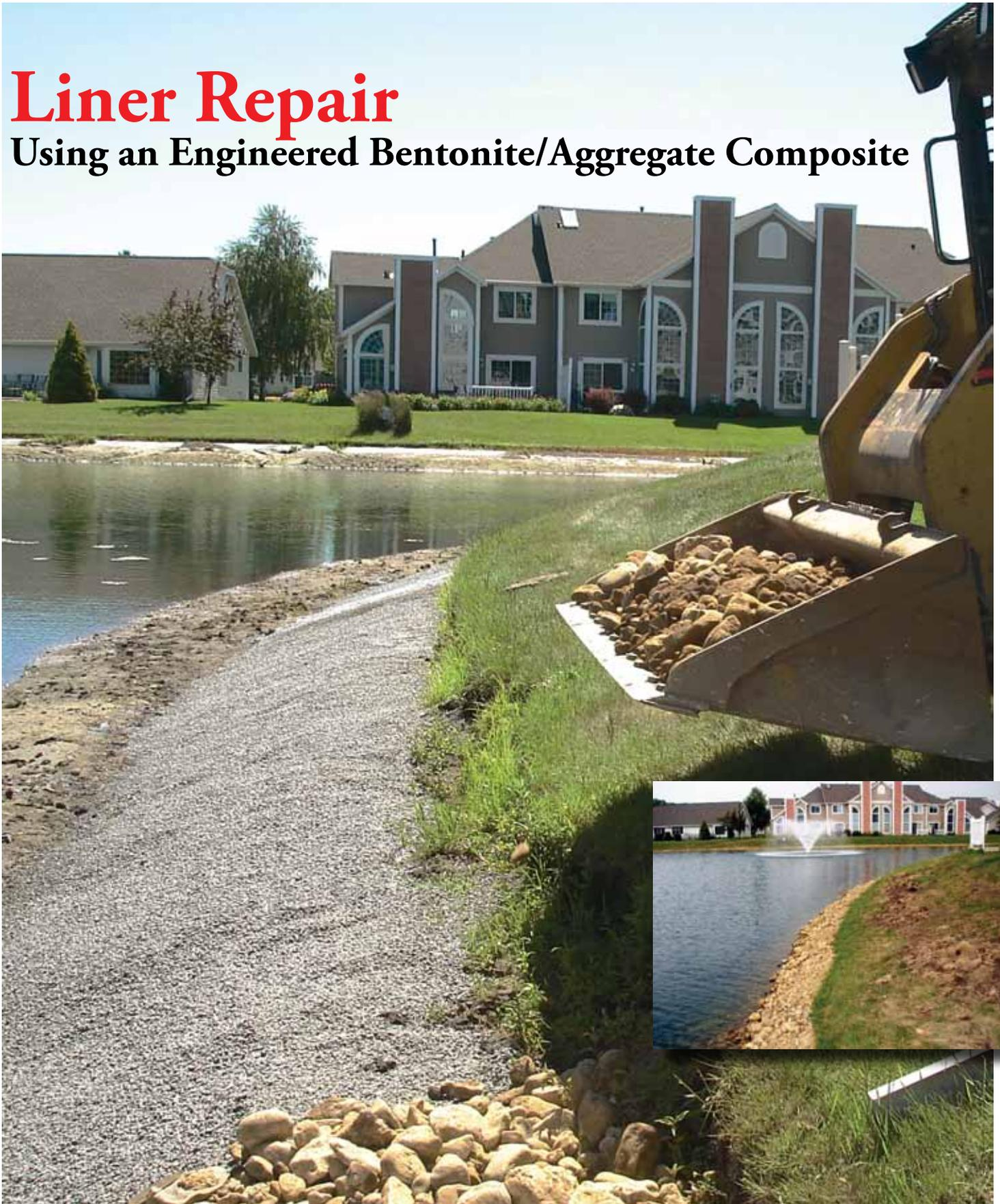
**Above:** Placement of armor stone (for erosion protection, site safety, and visual appeal) atop the pre-hydrated bentonite/aggregate composite. **Inset:** Waterford Lake, post-liner repair. Note water level has returned to desired/desired level.
