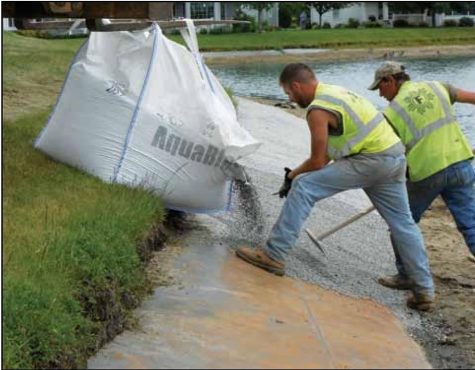
Placement of the bentonite/aggregate composite directly out of a shipping tote (note suspension of the bulk super sack on a long-reach forklift).
