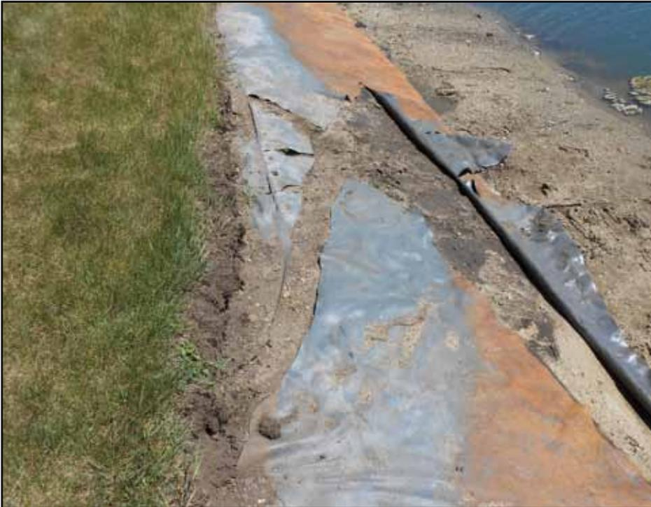
A typical cut in the HDPE liner impacting an approximately 2' x 6' area of the basin's shoreline edge - probably caused by a combination of UV exposure, ice damage, and age.
