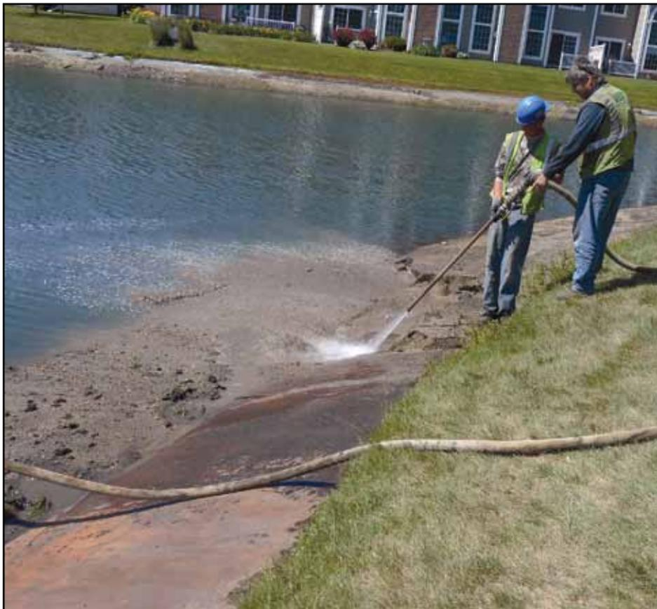
**Contractor removing up to 12-inches of cover sand/soil atop the compromised HDPE liner using a power washer at moderate pressure.**
