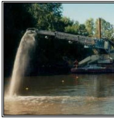
Photograph 1. Product applied using barge-based conveyor.
