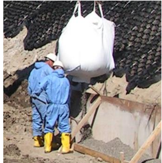
Figure 2. Placement of AquaGate+Provect-IRM
