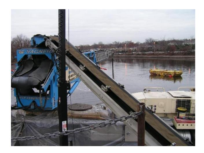
To improve control, placement is monitored with a computer system that essentially allows the operator to "paint" a target area at a uniform rate, collecting data on placement rate, based on feed rate and belt speed. This combination provides the operator with a significant amount of control over both the thickness of the layer, based on application rate (lb/SF of material from the belt). The photo to the right shows the control system used by the operator to track placement.
