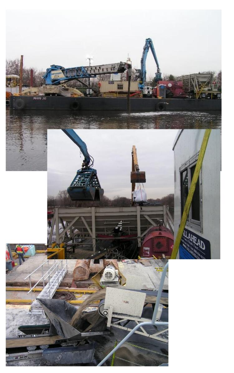
As noted below, the Telebelt receives material from the dual hopper feed system via a belt and interim mixing hopper. The top photo on the right shows the upper portion of the transfer belt where the samples of material were taken, as follows:
