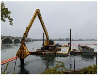
placement in the river. The target cap thickness was 12-inches.
