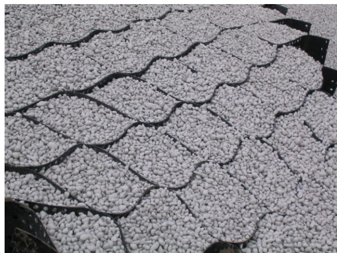
Close-up View of AquaBlok in Geocell
