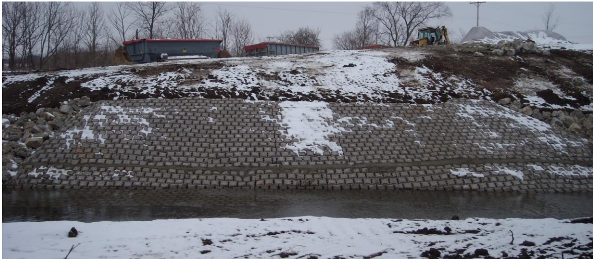
Overview of Completed Slope Repair/Stabilization with AquaBlok Landfill Cap Seal / Repair
