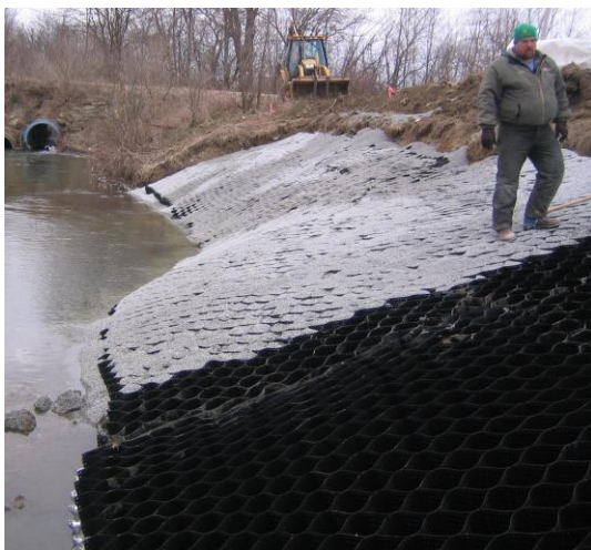
Overview of AquaBlok in Geocell on Slope
