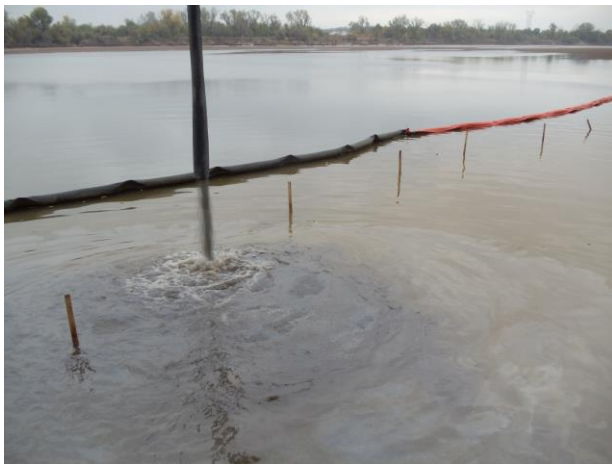
Above – Close-up of Telebelt Material Placement
