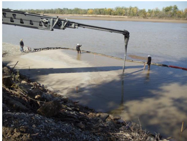
Above – Placement of AquaGate+Organoclay
