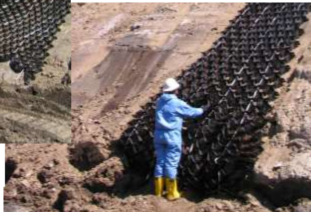
Below: Installation of Cellular Slope Stability Material (Geocell)
