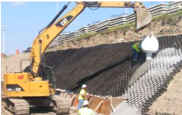
Above: AquaBlok Placement into Cellular Slope Stability Material
