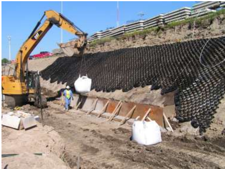
Above: AquaGate Placement into Form at Base of Slope
