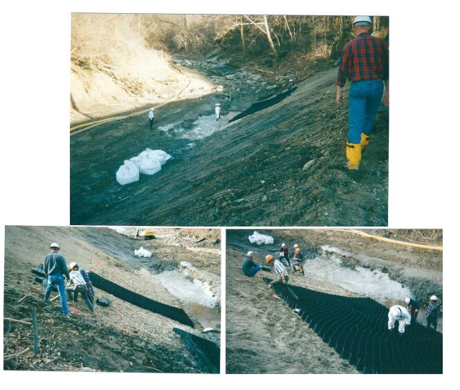
**Method of AquaBlok Placement:** Material placed directly from Supersacks suspended from a shore-based excavator (shown on previous page).
