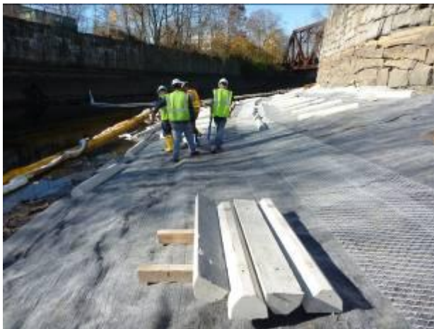
Concrete curb stops were placed on the RCM as anchors.
