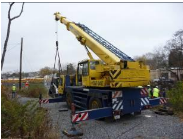
Materials were lowered into the canal with a crane.
