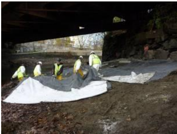
RCM was placed along the slope (by hand).
