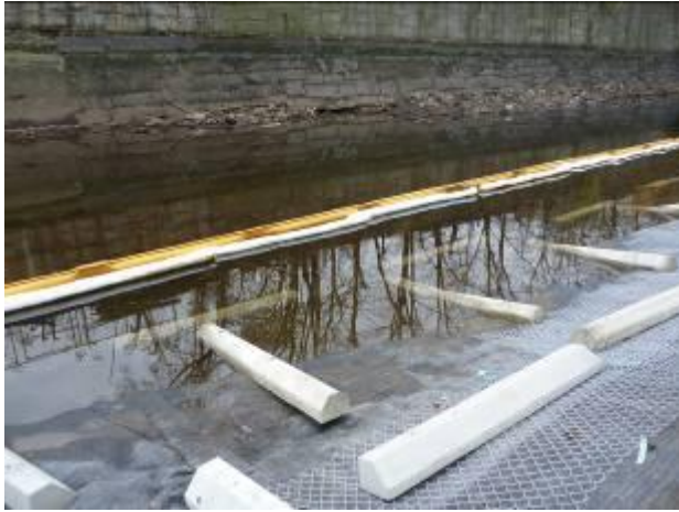
One continuous length of boom encircles the site.
