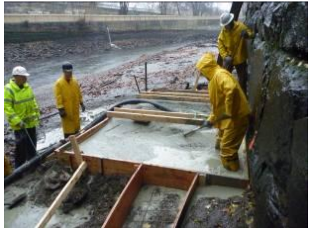
Poured concrete for upstream anchor strip pad.
