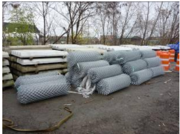
Materials: Concrete curb stops and chain-link fence
