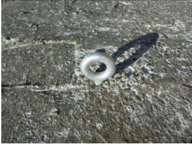
Eyebolts set into anchor strip.
