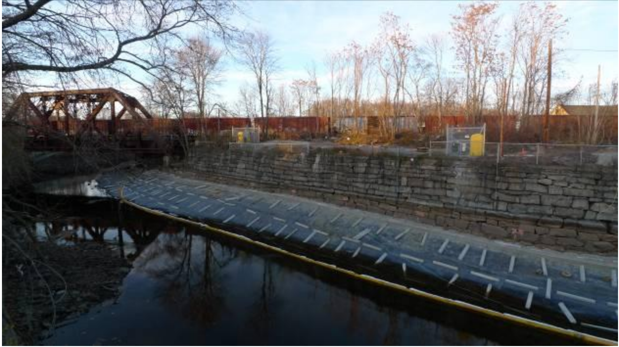
Pawtucket Canal Site – post construction (cap and anchor strip).
