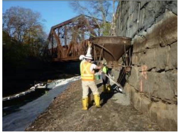
Aquablok was placed along the toe of the canal wall.
