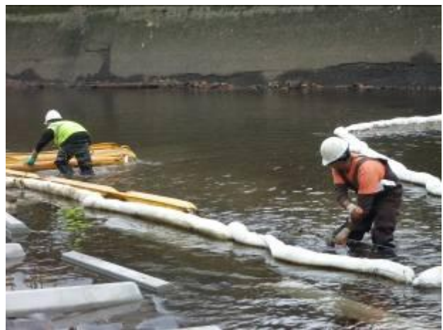
The hard boom and absorbent boom were adjusted.
