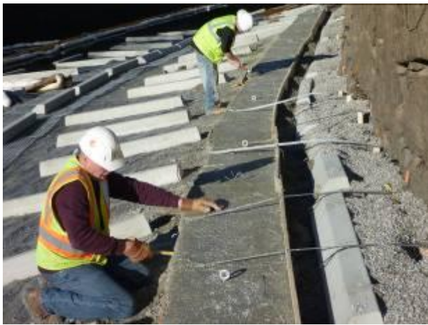
Removed forms for anchor strip.
