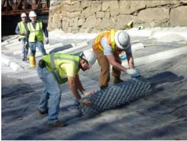
RCM seams parallel to the wall were covered with fencing.
