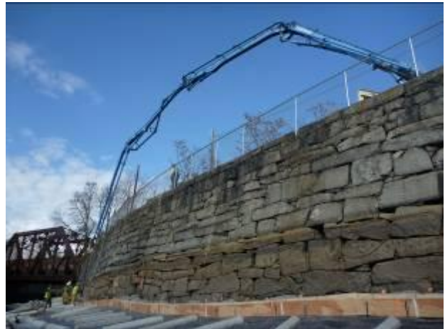
Poured concrete for anchor strip with a pump truck.
