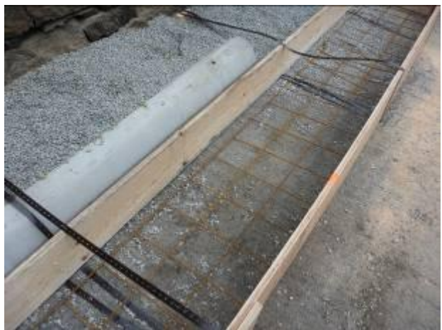
Completed anchor strip form.
