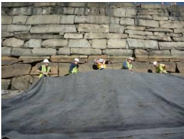
The placement of the RCM was adjusted as needed.
