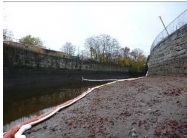
Downstream end of boom/cap installation area.
