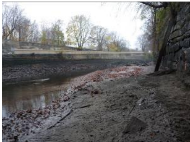
Upstream end of boom/cap installation area.
