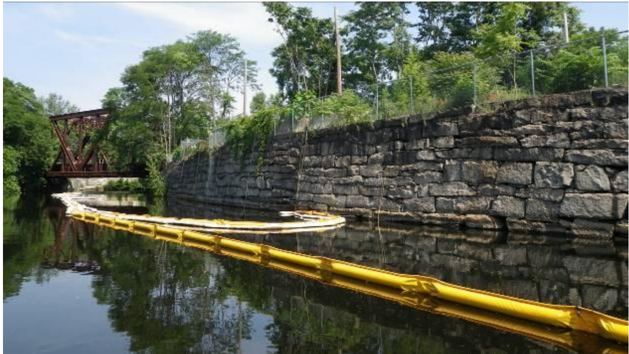
Pawtucket Canal Site – prior to construction.
