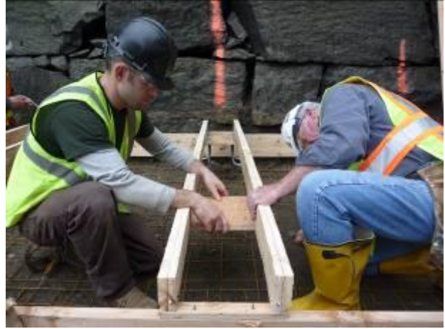
Set bolts in the pad for the Gunderboom end seal apparatus.
