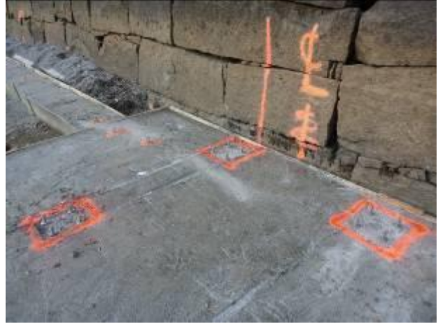
Bolts and eyebolts set into anchor strip pad.
