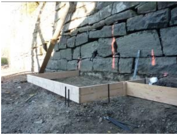
Form created for upstream anchor strip pad.
