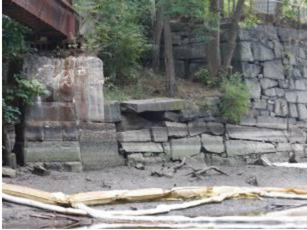
Prior to cap installation, debris removal occurred.
