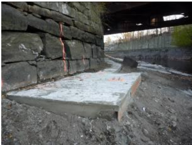
Completed upstream anchor strip and pad.
