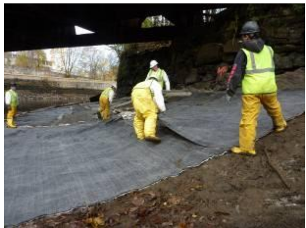
Seams between RCM sections were overlapped by at least 1 foot.
