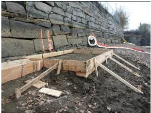
Form created for downstream anchor strip pad.
