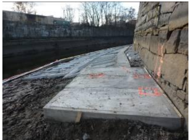
Completed upstream cap, anchor strip, and pad.
