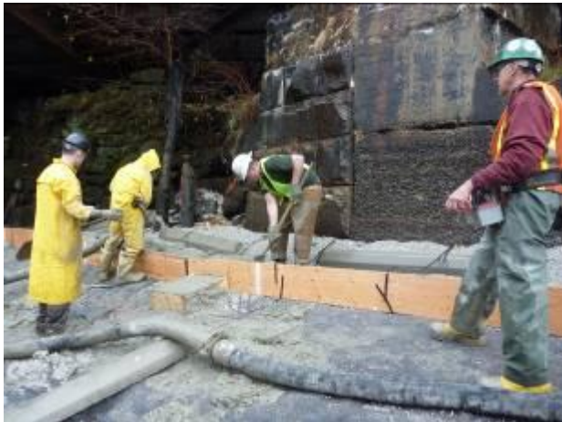
Poured concrete for anchor strip.
