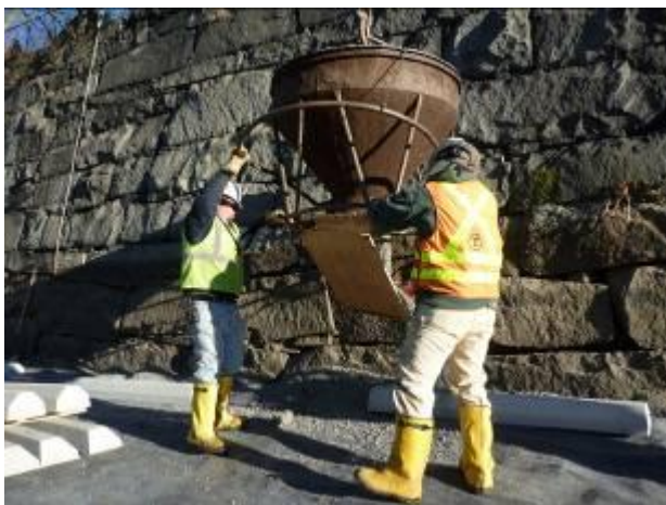
Aquablok was placed above the RCM along the wall.
