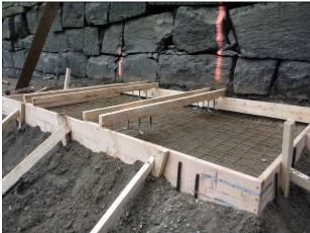
Completed anchor strip pad prior to concrete pour.
