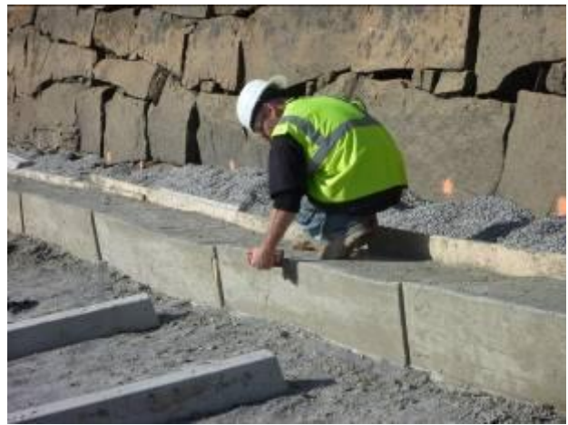
Smoothed the edge of the anchor strip.
