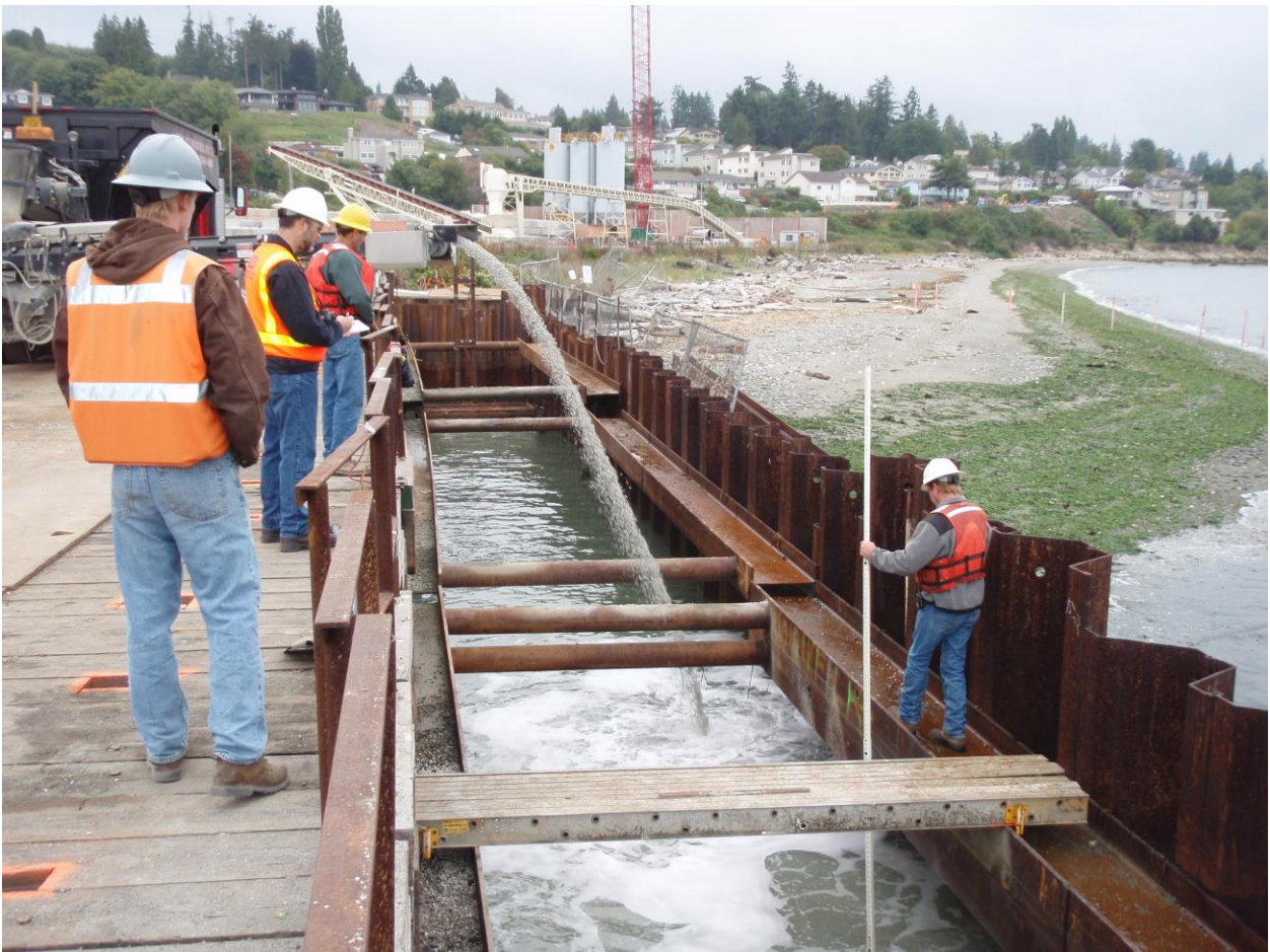
Placement of low permeability pipe capping material
