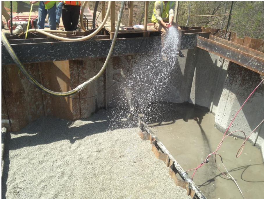
Hydrating AquaBlok with Freshwater after Installation
