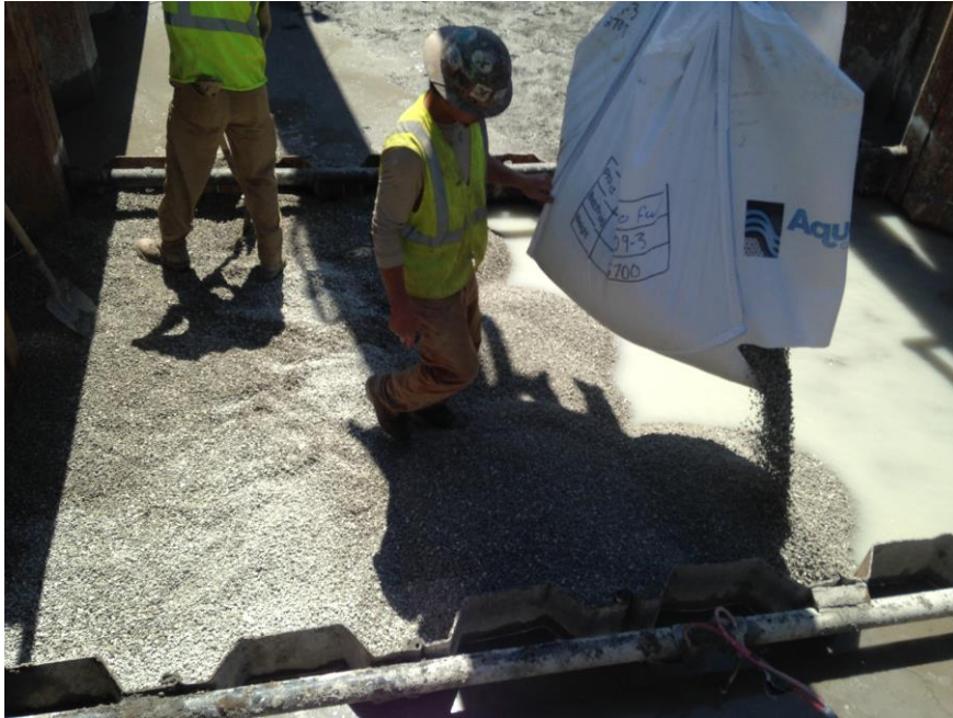
Placement of AquaBlok was performed in lifts directly from bulk bags
