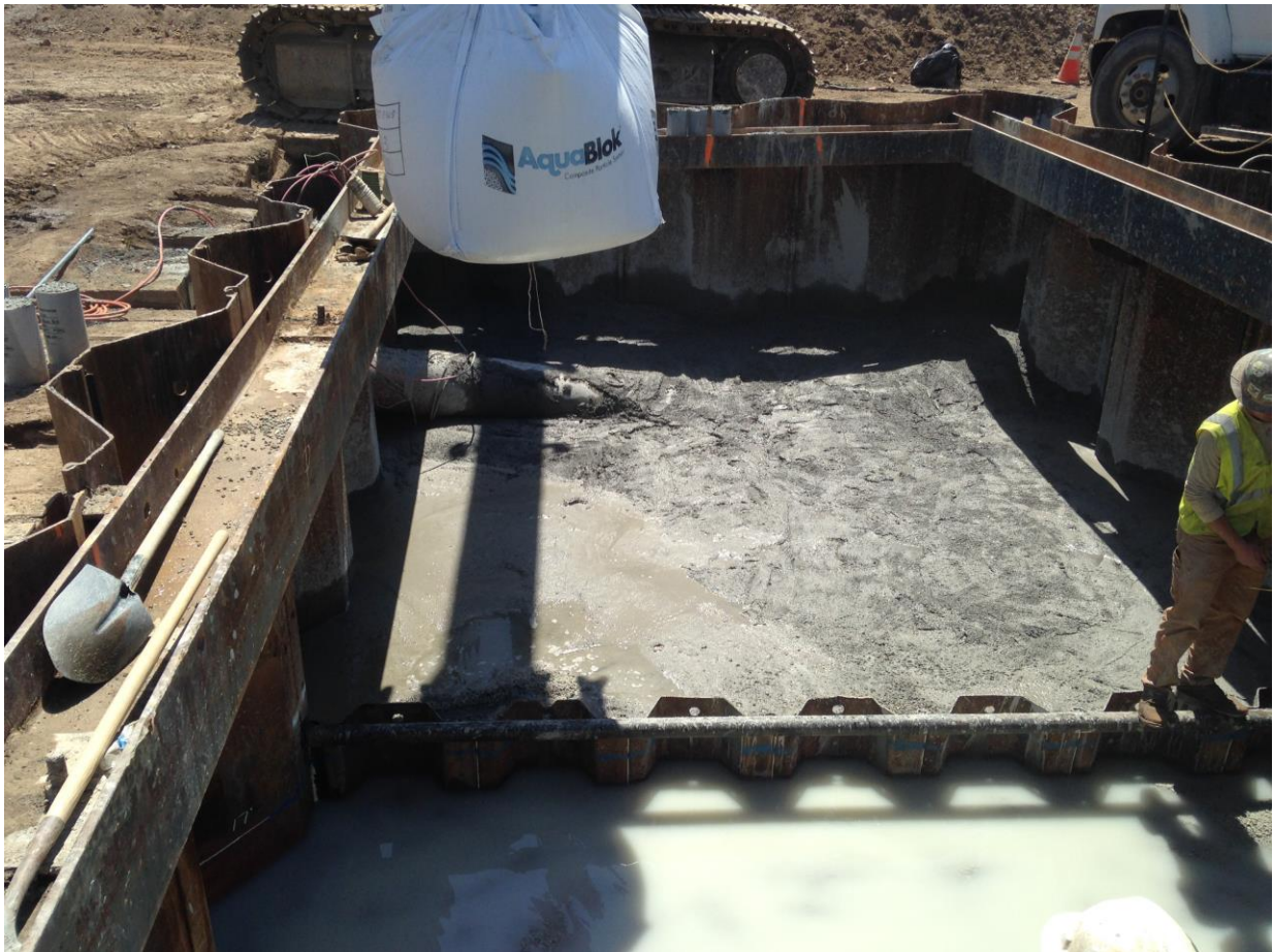
Placement of low permeability pipe capping material
